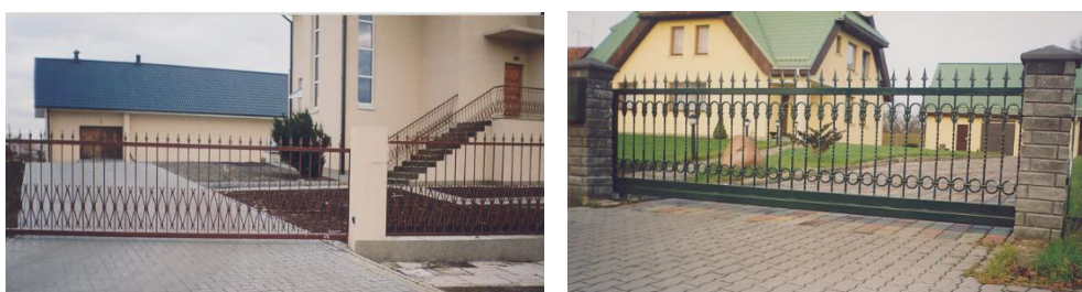
Figure 2. The gates erected to restrict transport and pedestrian traffic
